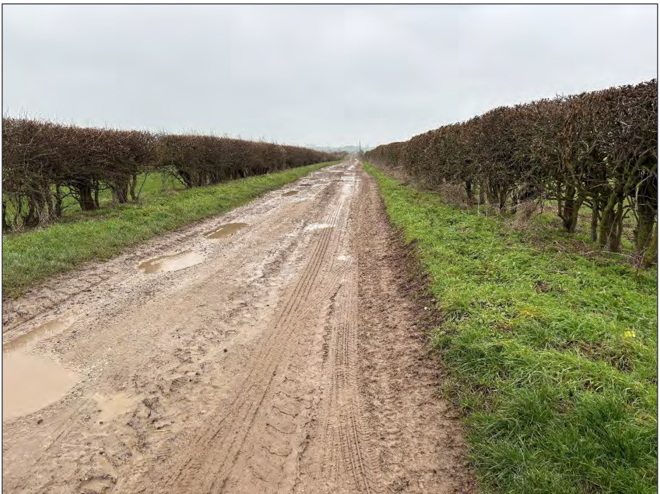
Figure 2.1 Typical Road Condition
