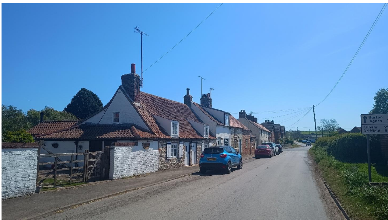
Plate 20: View looking south south-east towards the Grade II listed Buttercup Cottage (1162406, centre left) and looking in the direction of the site.
