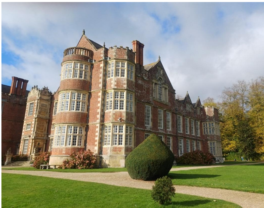
Plate 26: East and south facing elevations of Burton Agnes Hall. The projecting Library windows on the 2 nd floor have views south and east. The Long Gallery is on the 2 nd floor, adjacent to the Library on the east (right) elevation.
