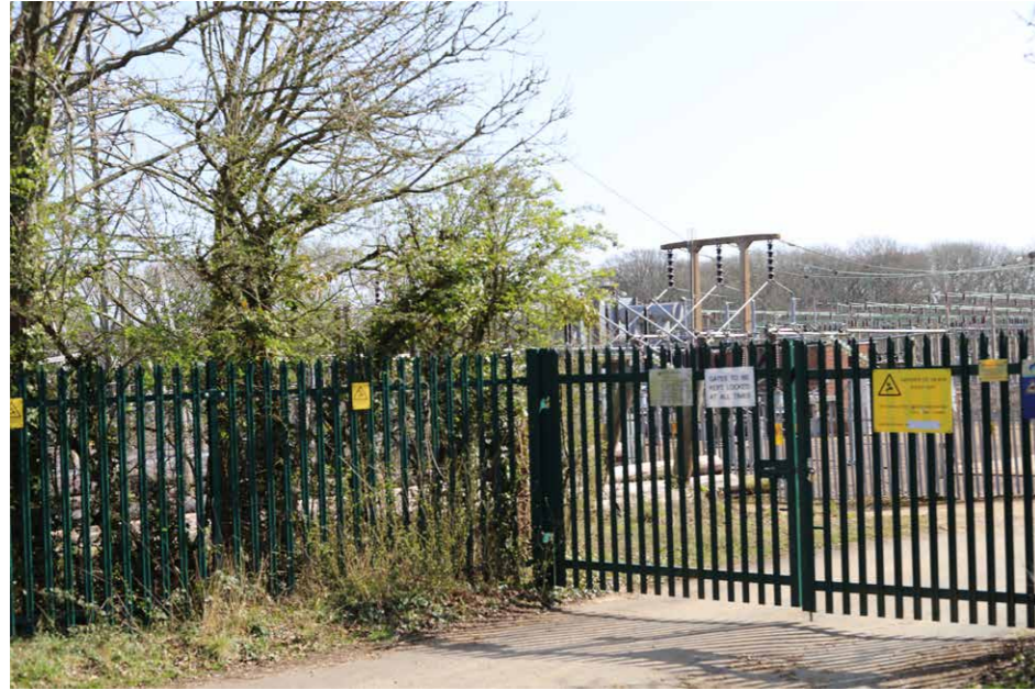
VP3a Staplers Road, positioned 230m NE of VP3
