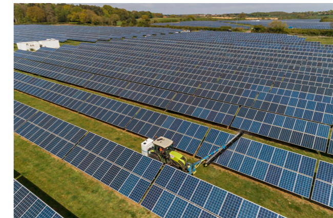
Example of Site Cleaning Techniques
