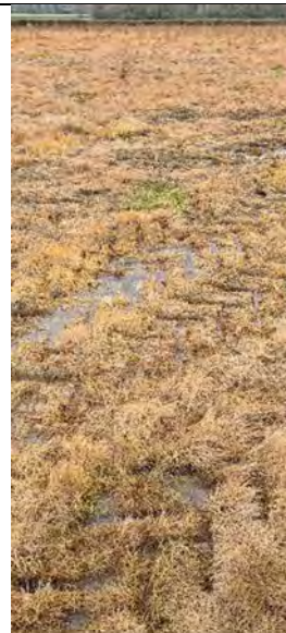
Waterlogged/Surface water land at BRID 11, 14, 15 & 20
