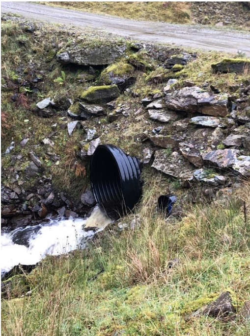
Plate 10.5. Culvert installed to allow for the continuous flow of Allt Mhadaidh. Watercourse flows east to west. Plastic culvert >1m wide with a 2m wide watercourse. Boulders and cobbles in Riverbed. NGR NN 09922 15111. Culvert view (left) downstream (right).
