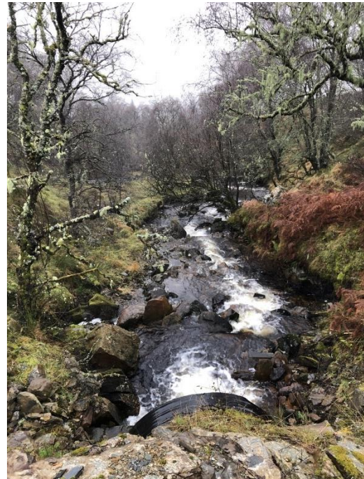
Plate 10.5. Culvert installed to allow for the continuous flow of Allt Mhadaidh. Watercourse flows east to west. Plastic culvert >1m wide with a 2m wide watercourse. Boulders and cobbles in Riverbed. NGR NN 09922 15111. Culvert view (left) downstream (right).
