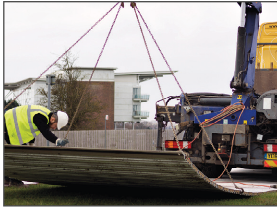
Plate 6.2 - Installation of Temporary Trackway
