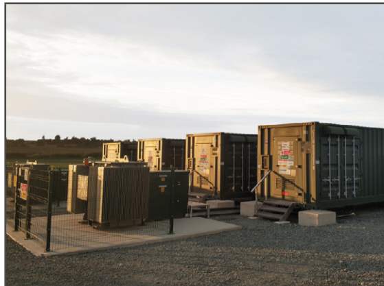
Plate 6.8 - Typical Battery Energy Storage System
