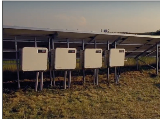
Plate 6.4 - Typical string-inverter units
