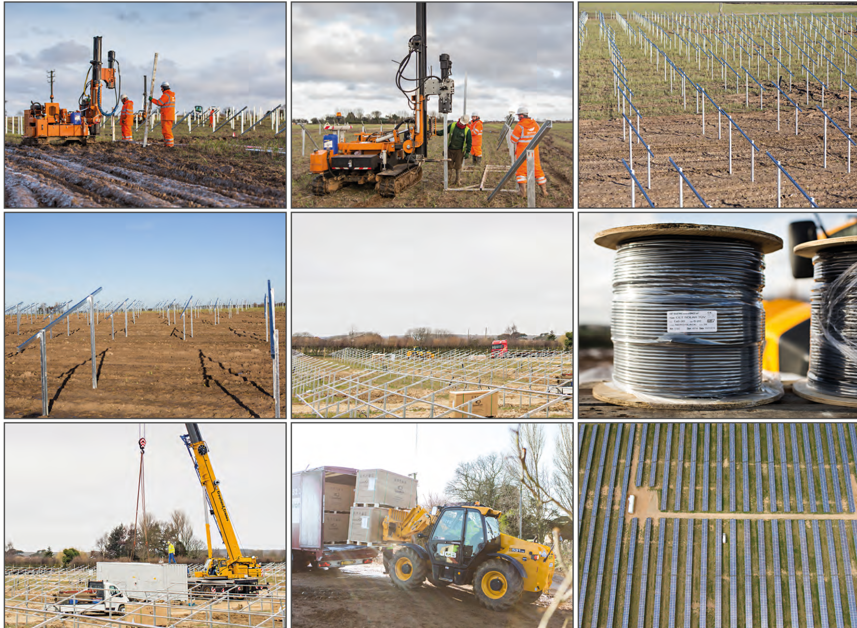
Plate 8.1 - Photographic Sequence of Construction Process
