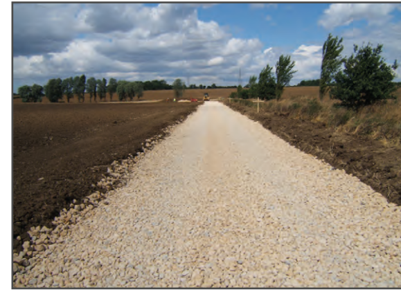
Plate 7.2 - Typical New Site Access Track
