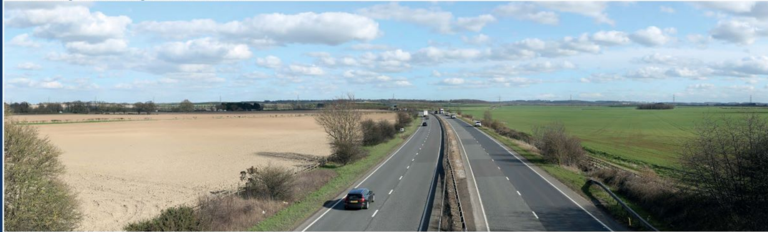
Existing view looking east from the A14
